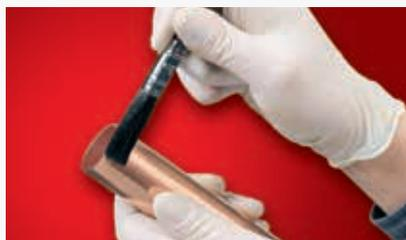
2. Insert the tube into the fitting until it reaches the tube stop, using a twisting action to ensure the spread of flux. Ensure the tubes are correctly lined up and adequately supported – otherwise distortion or cracking may occur when at brazing temperature.
