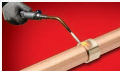
If the complete ring of solder does not appear on heating, apply additional flux to the mouth of the socket and end feed the joint with our N165 (Copper coloured) or N166 (Brass coloured) cadmium-free silver brazing alloy, or an equivalent to the compositional requirements of BS EN 1044 AG103 (formerly BS 1845 AG14).
