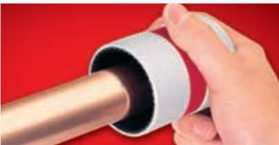
**3.** Clean the inside of the fitting socket and the outside of the tube with a Yorkshire cleaning pad, fine sandpaper or steel wool.
