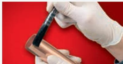
**2.** Insert the tube into the fitting until it reaches the tube stop, then wipe off any excess flux. Heat the assembled joint until a complete ring of solder appears at the mouth of the fitting.
