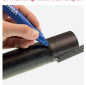
The required insertion depth must be marked on the pipe or the press fitting (the latter for fittings with pipe ends) in order to guarantee a safe and proper joint. The pressing operation behind the bead is of crucial importance for the tensile strength.
