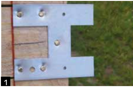
1 Fix the stiffeners at 300mm centres.
