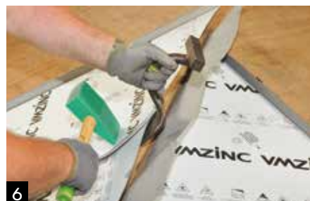
The seams are again flattened.
