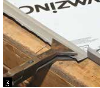
3 Fold back standing seam.
