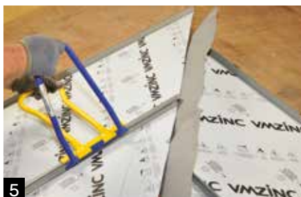
Panels on the other side of the hip are seamed up.
