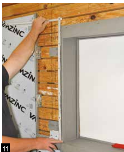
8 Jamb with reveal joint prior to installation.
