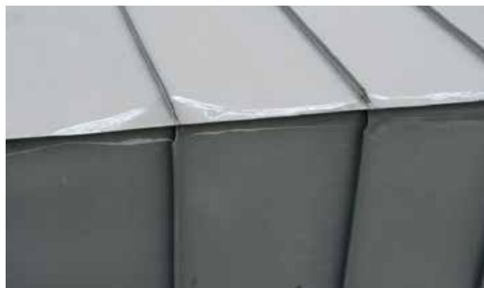
Staining resulting from partial removal of protective film.
