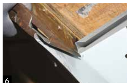
6 Finish fold on panel upstand.
