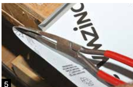
5 Create fold on panel upstand.
