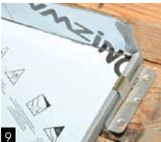
9 Install panel with sliding clips below the rooflight.
