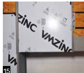
15 The next standing seam panel is installed with sliding clips.
