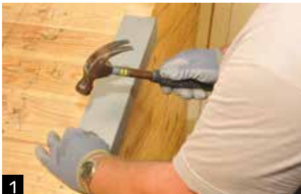
1 Install a zinc clip with nails leaving a 20mm space with the verge.
