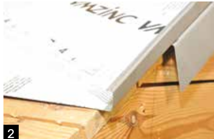
2 Position the standing seam panel.
