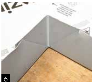
6 Position and then solder corner gussets.
