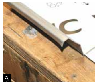
8 Cut back standing seam by 25mm. This enables a tab to be folded back prior to soldering above the rooflight.
