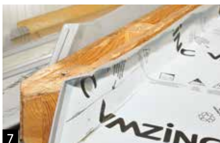
The hip batten is installed.
