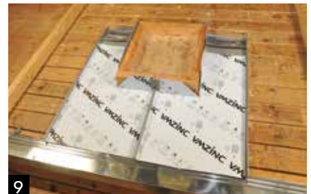
9 Alternative positioning of welted joint.
