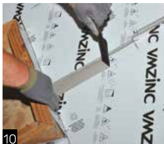
10 Peel back film on area to be soldered.
