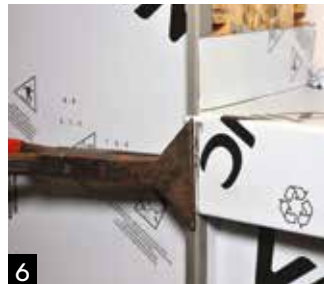
6 The sill is installed and the folded around the seam.
