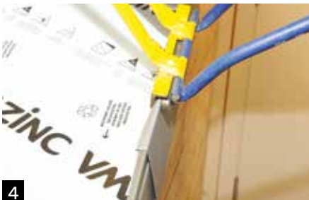
4 Crimp the standing seam at the verge.
