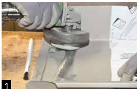
1 Fold 25mm hem on panel and remove patina 150mm further down panel.
