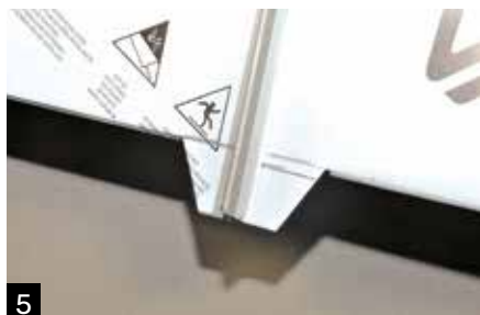
5 Fit the upper panels as per the eaves. (See page 12)
