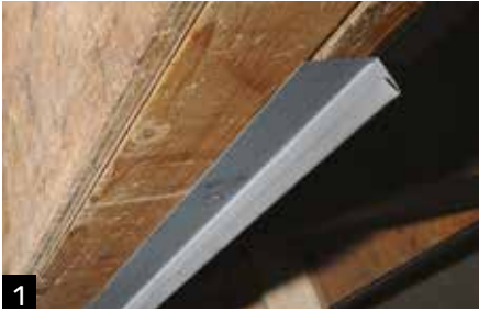
1 Fix a base flashing to the bottom of the soffit using screws.
