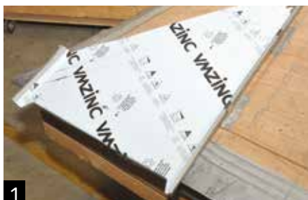
Panels are installed on the hip.
