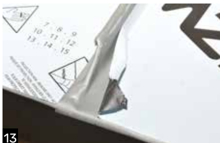
13 Completed eaves prior to film removal.
