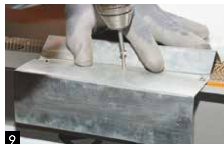
9 Fit clip for ridge flashing.
