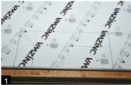
1 Mark out rooflight and include 100mm upstands.
