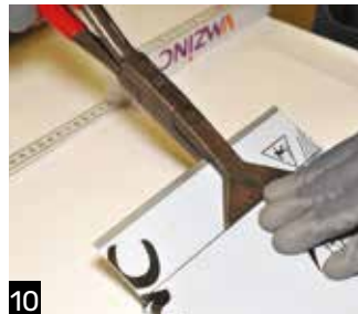
10 A standing seam jamb is made with a 50mm return for the top.
