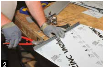
2 Cut away return fold on the profiles.
