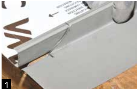
1 Mark the zinc with a template (80mm in length).
