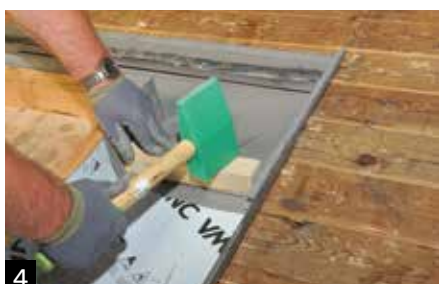
4 Complete double welt by gently hammering a wooden block onto the lower hem.
