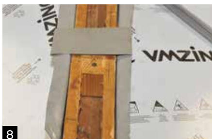
A zinc clip is installed prior to the hip flashing being fitted.
