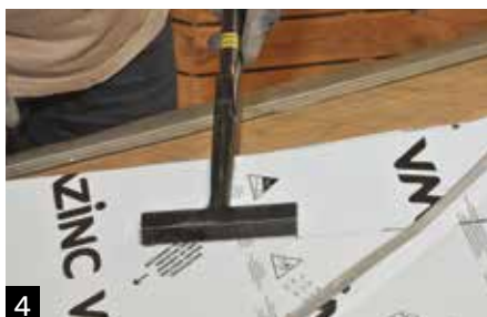
The panel is folded upwards.
