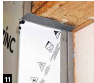
11 The jamb with the friction grip is installed.
