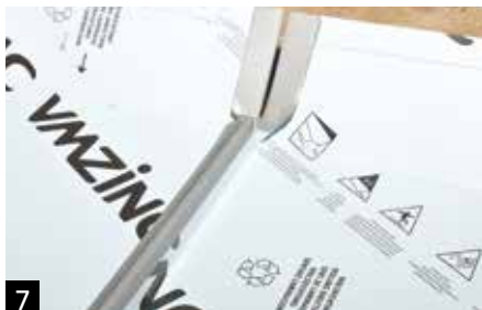
7 Seam panels together.
