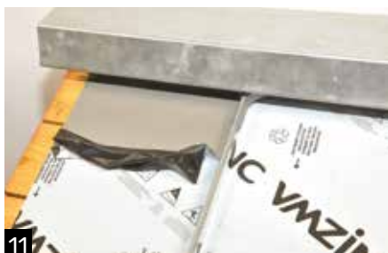
11 Do not partially remove film.
