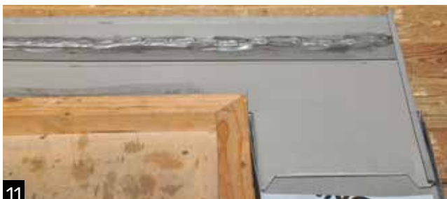
11 Back plate installed as a double welt.
