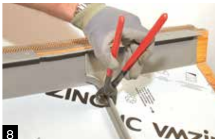
8 Fit saddle piece and pinch at seam.
