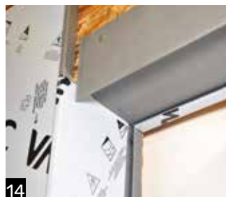
14 The head flashing is fitted using the friction grip and slotted holes for screws.
