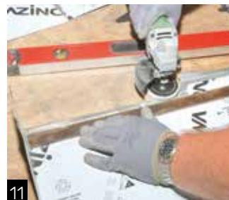
11 Remove patina on all areas to be soldered. This can sometimes be done prior to panels being installed.
