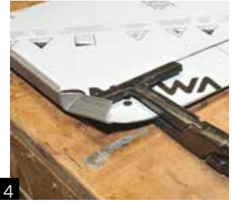
4 Create dog ear fold at bottom of rooflight.
