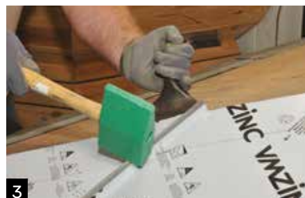
The seams are carefully flattened over 150mm.
