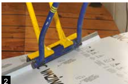
The seams are crimped beyond the hip.
