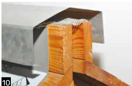
10 Insert ridge flashing.
