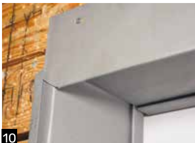
7 Jamb receiver strip installed and jamb measured.
