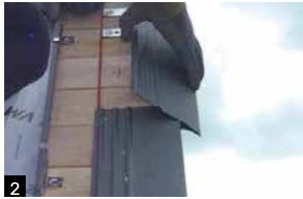
2 Fit the verge strip into the stiffener and fix with nails. The strips should overlap by 50mm.
