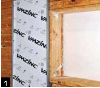
1 The 1st panel is installed aligned with the jamb.
