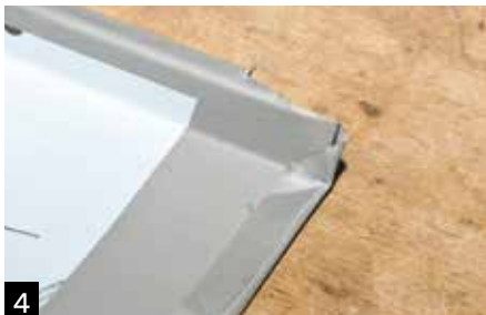
4 Create safety check at top of panel.
