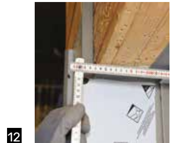
12 The head receiver strip is fitted and a measurement for the head flashing taken.
