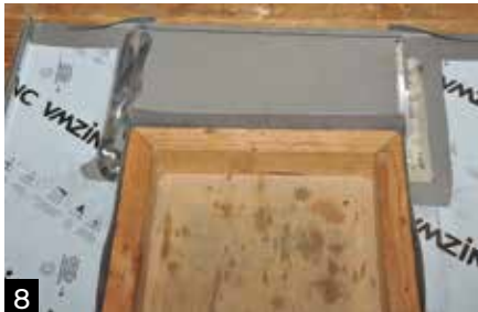
8 Solder back plate into position.
