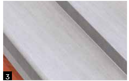
3 The standing seam panels are fitted in the normal fashion and by being hooked into the verge strip with a 30mm hem. The distance between the verge and the first seam must be at least 150mm but no more than 370mm.
