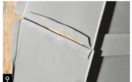
9 Fit adjoining flashing and turn up folds.
