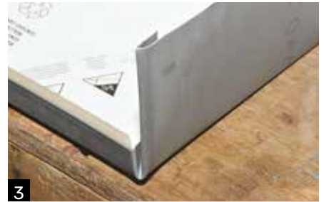
3 Create dog ear fold at bottom of rooflight.
