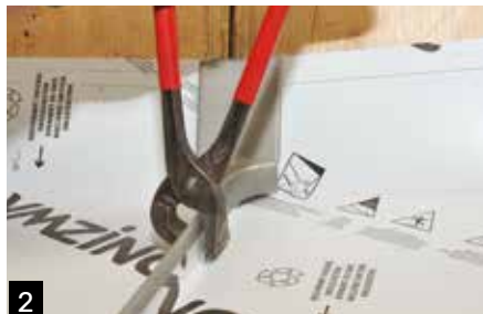
2 Pinch saddle piece into place.
