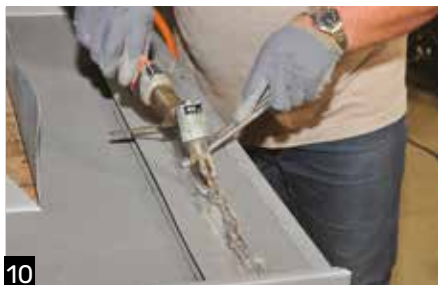
10 Back plate with soldered strip.
