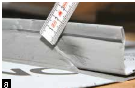
8 Mark the zinc at 15mm above the cut edge.
