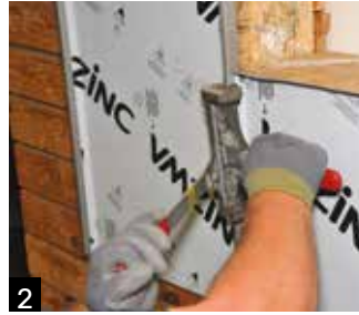
2 The panel below the window with a 15mm return is installed using a single lock.
