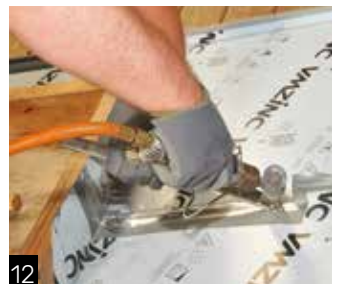
12 Solder panels together.
