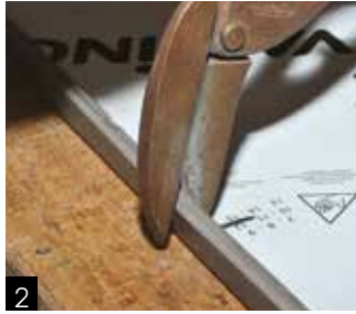
2 Cut back seam at 300mm from top of rooflight.
