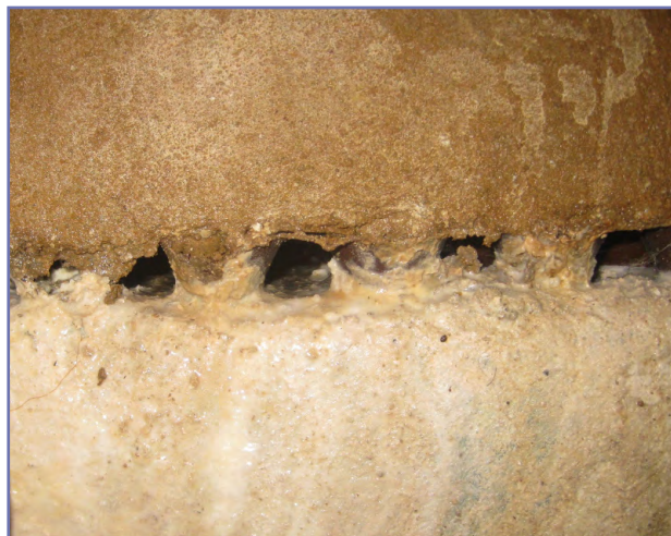
Figure 1: When free lime completely blocks a Type C system, leading to total system failure
