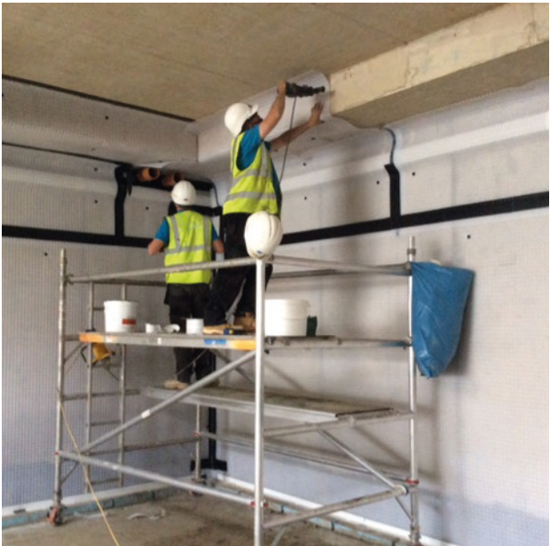
The Newton 508R that forms the air-curtain is neatly fixed to terminate at the soffit
