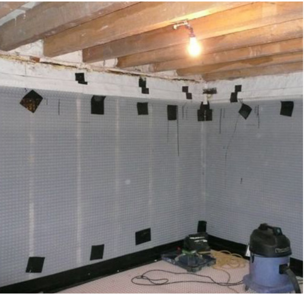
Newton PAC-500 System installed to a house in Derbyshire with very high levels of radon gas
