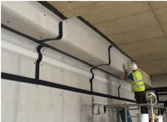
Case Study: Ground Gas Protection and Waterproofing: New-Build Mansion The Newton PAC-500 was the perfect solution for this large-scale new build basement project which included multiple swimming pools.
