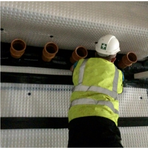
Penetrations through the membrane are carefully ‘double sealed’ to ensure gas tightness, ready for the trace-gas testing
