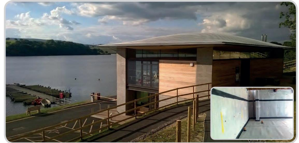
The pre-designed waterproofing system combined Type A (Barrier) and Type C (Drained) protection
