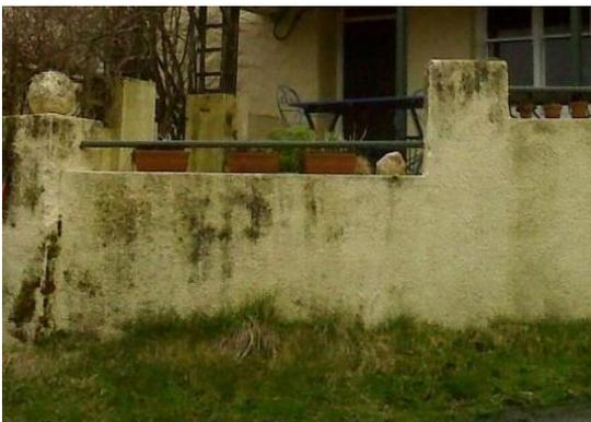
It is important to treat any surfaces affected by mould and fungal growth and to kill algae spores prior to redecoration. If spores are not properly treated then the growth can reoccur despite a quality redecoration.
