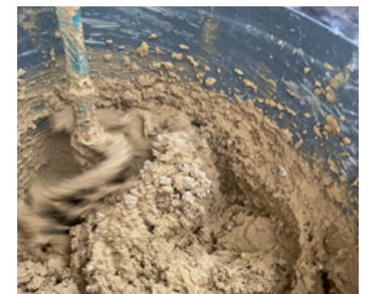
Direct addition to new Janus plaster mix for on-site recycling.
