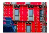
Far simpler than internal options Wraptite external air barrier system will maintain the envelope's integrity, with less building services and structural penetrations to be sealed, and less room for error.
