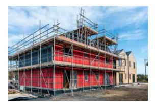
factory swapping from our usual airtightness board to flexible airtightness membranes between the modules. The cost of this was not sustainable so we needed to look for an alternative.
