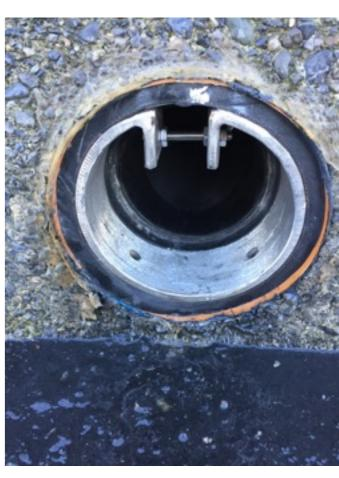
Insert CheckMate fully into pipe
