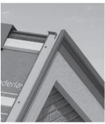
Fig. 27 – Interlock left and right hand trims
