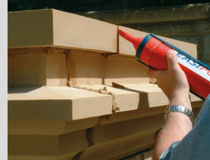
Easipoint mortar during installation.
