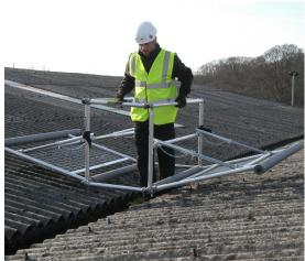
Valley-Walk is a mobile walking frame for one or two persons, designed to aid access along valley gutters and to provide mobile roof cover.
