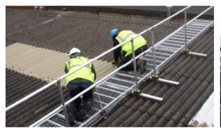
Board-Walk is an open mesh walkway that allows access from eaves to ridge whilst spreading the load on support battens to provide the user with a safer working position. The system is lightweight, easily portable and suitable for fragile roofs.
