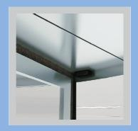
The internal ceiling is constructed with separate Silver Anodised Aluminium wedge shaped panels. These can be finished to match the door colour.
