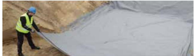
\*The geotextile should be selected according to specific site conditions. Typically, however, a 300g non-woven material will be suitable. Specialist advice should be sought if surrounding soil characteristics exhibit a high degree of fines/low infiltration capacity and/or there is a high risk of damage from ground contaminants.
