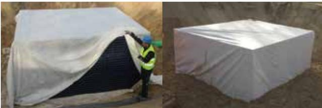
\*\*Typically, for large scale, deep installations a 1mm thick geomembrane is recommended and joints should be sealed using proprietary welding techniques, however specialist advice should be sought.
