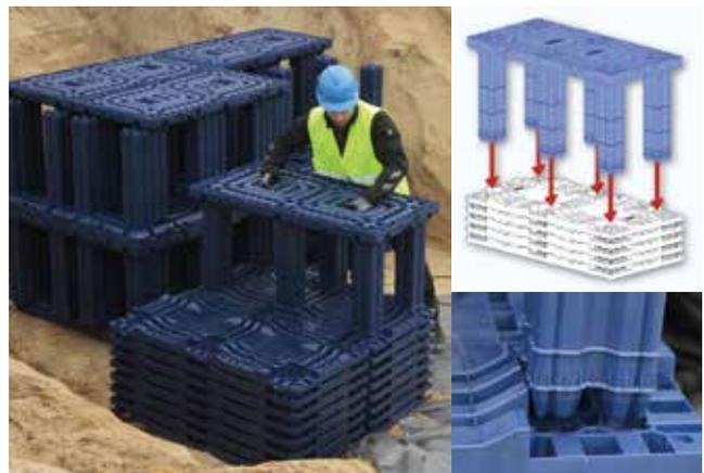
Slide and fix the assembled Column Units and Base Plates together using the integrated connectors to form the base of the structure.
