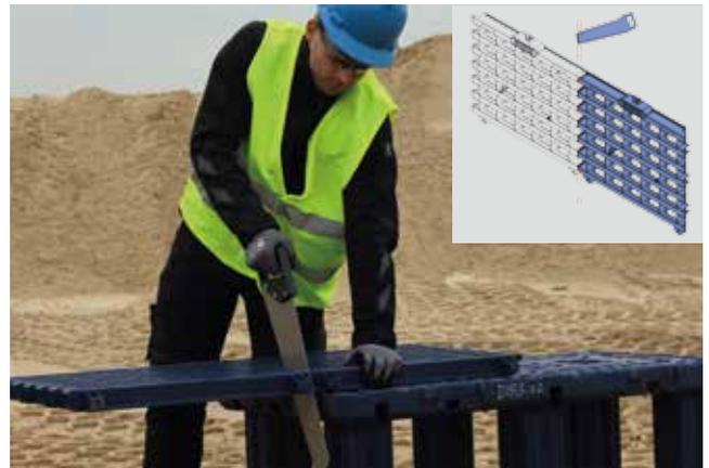
Only the non-cut edge of a Side Plate should be installed on a corner edge.
