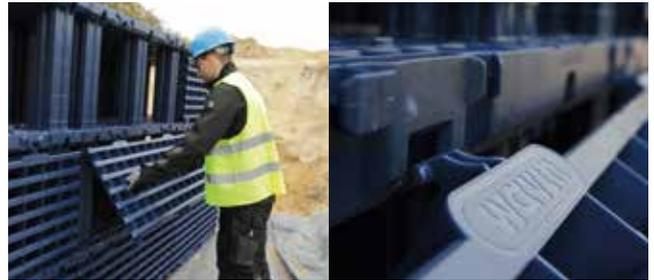
Where half of a Side Plate is required to be fitted next to a Connection Plate, then a full Side Plate will need to be cut in half (as shown below).
