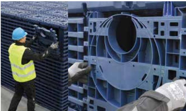
If using 160mm diameter pipe then assemble the pipe-stopper to the socket of the connection plate before attaching it to the main structure (as shown on the right). Alternatively, if using an adaptor fit this to the Connection Plate with self-tapping screws (not supplied).
