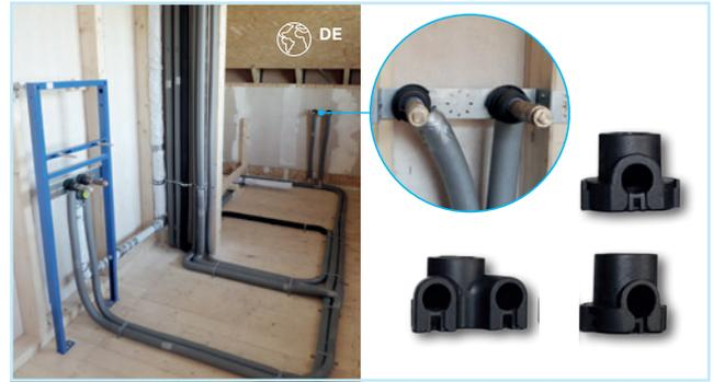
Figure 36: Sound insulation sets
