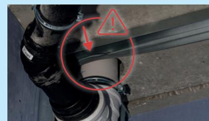
**Figure 41:** Avoiding contact with profiles
