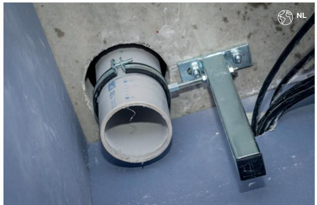
Figure 11: Fastening to elements containing mass
