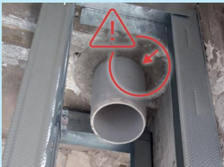
Figure 20: Forgotten structure-borne sound decoupling
