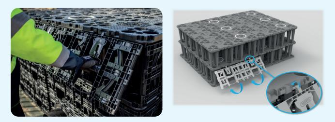
Repeat this step until all side panels are installed and the system is fully closed except at the location where the inlet and outlet must be placed.
