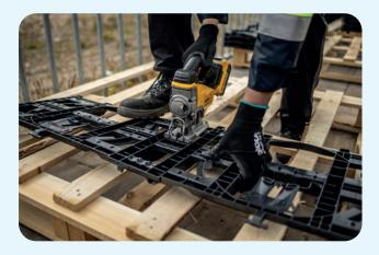
**Note 1:** In case of the need of a half sidepanel, the sidepanel must be cut.
