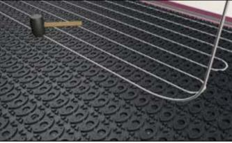
Return the first pipe run to the manifold.
