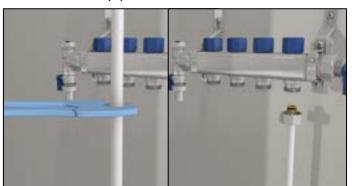
Connect all additional pipe runs to the manifold. Pressure test the system to ensure there are no leaks. Suitable expansion joints should be fitted at all door thresholds.
