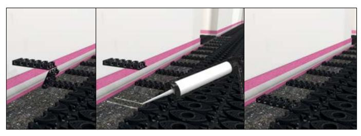
Profix® Clip-Rails can also be used in close proximity to the manifold to secure pipework at close centres prior to transitioning into the Profix® Panels themselves.
