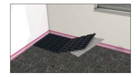
Stick down the panels as before to complete the first row, cutting the final panel in the row to size if required.
