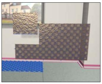
Commence laying the second row of panels by positioning the first panel in this row (with the male snapconnectors facing to the right and the front) parallel to the previous row. Ensure that the male snap-connectors along the front edge of the panel in the first row align with the females in this panel. Press the panel down to engage the snap-connectors and to fully adhere the panel to the floor.
