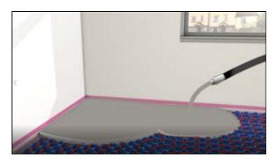
The screed should be levelled to the required depth using a levelling rake and/or smoothing trowel. The surface finish can be improved using a spiked roller.
