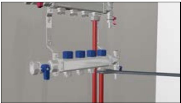
Return the first pipe run to the manifold.
