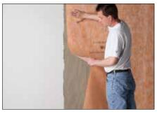
**Schlüter®-KERDI** is a crack bridging waterproofing membrane of soft polyethylene with a special fleece fabric laminated on both sides for effective anchoring in the tile adhesive.
