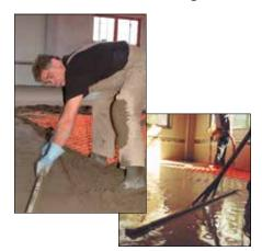
Prior to installing the screed, the seal of the heating system must be tested under pressure. However, the system may not be heated during the installation and curing process of the screed. For further information on filling and venting and a pressure test report, please refer to the Appen-
