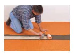
Schlüter®-DITRA 25 is a polyethylene membrane with cut back square indentations and an anchoring fleece laminated on the underside. In conjunction with tile coverings, Schlüter®-DITRA 25 provides waterproofing, vapour pressure equalisation for back side moisture and uncoupling. Joints and wall transitions are sealed with the seaming tape Schlüter®-KERDI KEBA, using the sealing adhesive Schlüter®-KERDI-COLL-L.
