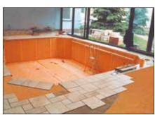
The surfaces of areas such as public showers, swimming pool surrounds and barrier free bathrooms must be constructed as bonded waterproofing assemblies. The following products of Schlüter-Systems may be used as supplements:
