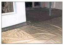
Installation of separating layer
