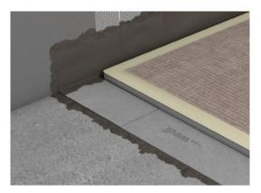
Now fold the sealing corners into the 520 sealant, and apply another layer of sealant on top, ensuring to fully embed the corners as well.
