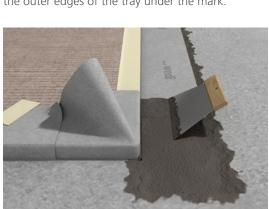
Apply wedi 520 sealant to the adjacent surfaces. Fold the tape into the 520 sealant, then apply another layer of sealant on top, ensuring to fully embed the tape.
