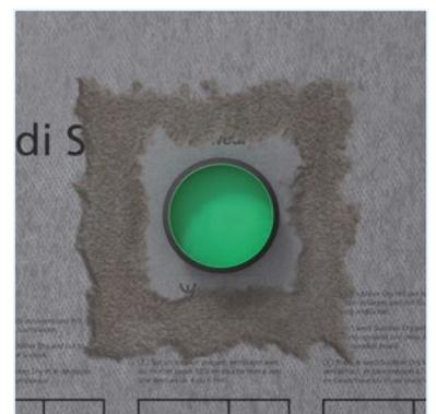
Seal pipe penetrations with wedi Tools sealing gaiters and wedi 520 flexible sealant.
