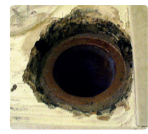
When a pipe is sheared close to a surface, with no stub or spigot
