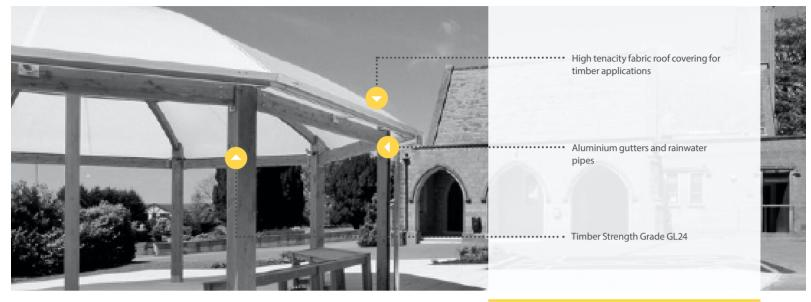
A great advantage of glulaminated (glulam) timber is that it can be manufactured in a wide variety of configurations. It is well known for excellent strength and durability, lending itself to architecurally pleasing solutions.
