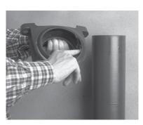
2. Push coupling over the end of pipe/ fitting, ensuring the central register is abutted against the spigot edge evenly. If the coupling is eared, fix to wall using anti-corrosion coach screws or similar.
