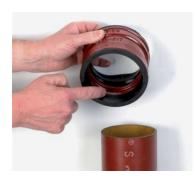
1. Apply a small amount of jointing lubricant on the lip of the rubber gaskets at both ends to ease insertion of pipe/fittings.
