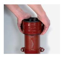
2. Push joint over the end of pipe, ensuring the central register is abutted against the spigot edge evenly.
