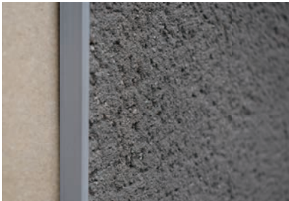
ProBead in ‘Dolphin’ creating sharp details with ProRend render
