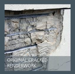
The repetitve expansion and contraction of the EML meshing in different temperatures had cracked the render around it. Water could then penetrate the cracks, saturating the render causing it to crumble when frozen.
