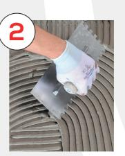
Using a 6mm notched trowel spread a substrate compatible flexible tile adhesive over the substrate.
