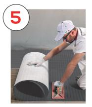
Lay the next sheet of membrane taking care to align it with the previous one, without overlapping. Align the square studs to enable the cable to be installed. Repeat previous steps until the room is covered in membrane as required.
