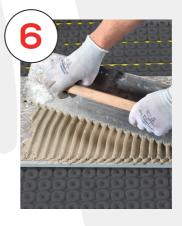
With the heating cable installed, you can apply a suitable adhesive (or self-levelling compound) and start laying the flooring. With the flat side of the notched trowel, fill the studs and cover the membrane with a suitable adhesive. Take care to cover the heating cable, the end cable connection and the floor sensor in the floor. Apply the adhesive with a notched trowel, appropriate to the tile size and lay the flooring.
