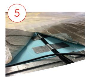
**5.** Install the floor sensor in the conduit, tape the conduit to the insulation and tape the end of the conduit to ensure the sensor does not protrude. Ensure that the end of the sensor is equidistant between two loops of heating cable.
