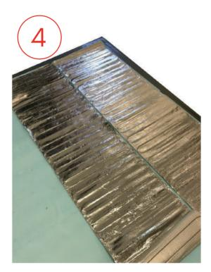
**4.** When you reach the end of each strip of heating mat, carefully cut the mat by cutting the mesh and foil (NOT THE HEATING CABLE) and turn the mat, positioning the next piece beside the first.
