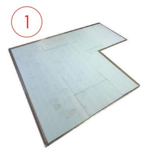
1. Before installation, the subfloor must be clean, dry, level and all protrusions removed. Lay the Gaia-XPS insulation, ensuring the whole floor is covered. To prevent movement, fasten with tape, DO NOT use any type of spray adhesive to stick the insulation down.
