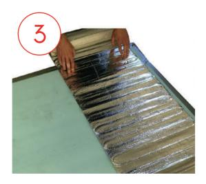
**3.** Place the cold tail of the mat at the connection point and begin to lay out the heating mat, leaving a minimum 20mm gap between the foil on each run and staggering heating cable loops. You may need to chase the connection leads into the Gaia-XPS insulation to ensure the depth of the system isn't increased.
