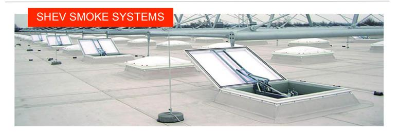
For the essential flow of smoke and hot air out of a building in the event of fire - certified to EN12101-2
