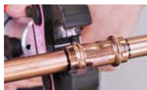
9. Align jaws squarely on the fitting
