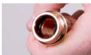
6. Ensure the O-ring is seated
