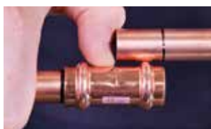
7b. Check the depth mark
