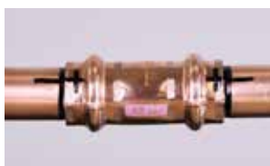
11. Mark the completed joint
