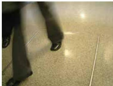
Aluminium floor access covers for use with flexible floor coverings
