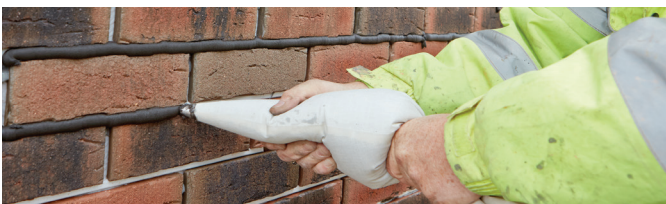
Applying mortar
