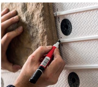
3. Before the stone slips can be glued to the backer panel, some of the horizontal ribs will have to be cut away to make room for the larger slips. Offer up the slips to the panel and draw lines to indicate the ribs to be removed.
