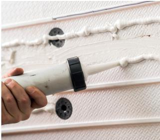
**6.** Apply a generous bead of high grab adhesive  $\frac{3}{4}$  of the way up each standard course, ensuring the fastener head is covered. For a double or triple course sized slip, use 2 or 3 beads of adhesive respectively.
