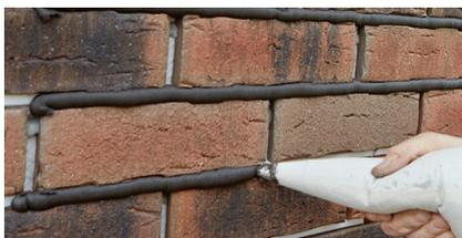
4. Specially formulated mortar is then piped into the brick joints.
