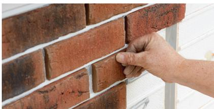
3. Brick slips are pushed into place leaving 8-12mm perpendicular gaps between bricks.
