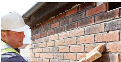
6. Once the mortar has set but not dried the brickwork is brushed to finish.
