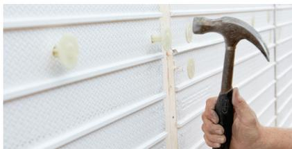
1. System backer panel arrives as one composite sheet. The panel is fixed to the substrate using appropriate fixings.
