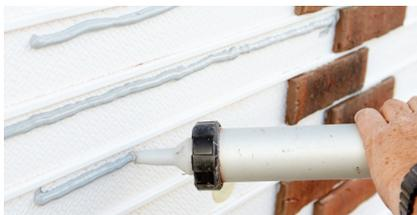
2. Permanent bonding adhesive is gunned in continuously towards top of course.
