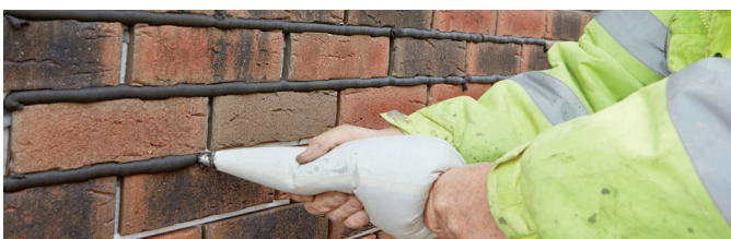
Applying mortar
