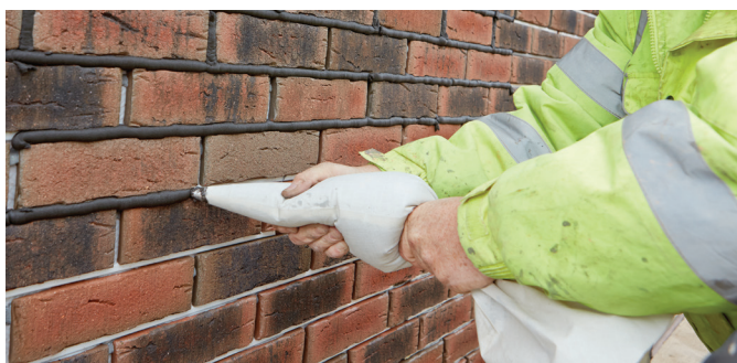
Applying mortar
