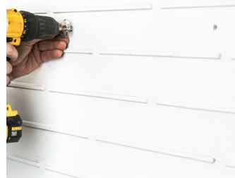
1. The ribbed backing panel is fixed to the substrate.
