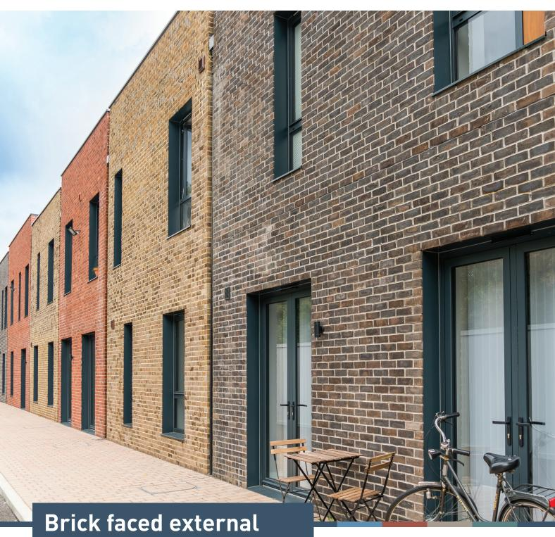
Brick faced external wall insulation system
