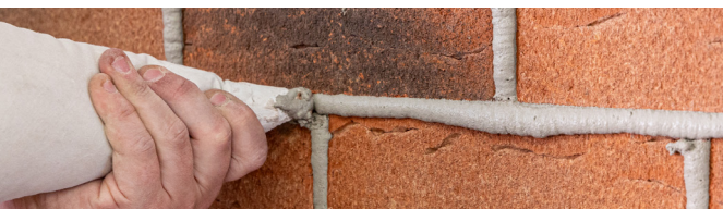
Applying mortar
