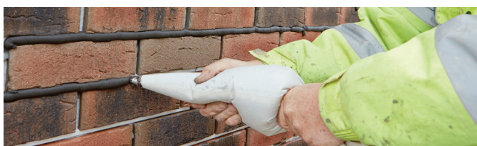
Applying mortar
