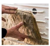
**7.** Apply stone slips between ribs ensuring each piece is firmly seated with full contact to panel.
