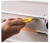
**4.** Carefully cut away the ribs to create a flat surface for the larger stone slips.
