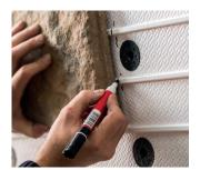
1. The stone slips come in three different heights representing one, two or three courses on the ribbed backer panel. Place the slips on the ground to determine desired layout. This is generally a process of trial and error, until you are satisfied.
