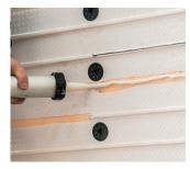
**5a.** Seal the panel where the ribs have been removed by applying adhesive over the "scar".
