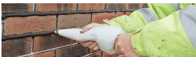
Applying mortar
