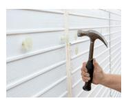
1. The ribbed backing panel is fixed to the substrate. (Fixings vary according to substrate.)
