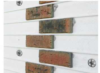
2. Brick slips are attached with permanent bonding adhesive.
