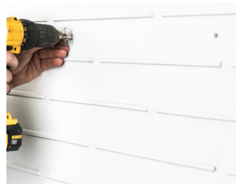
1. The ribbed backing panel is fixed to the substrate. (Fixings vary according to substrate.)
