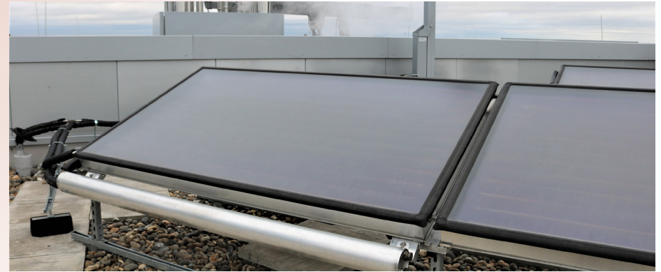
| Solar thermal preheat for gas-fired water heating
